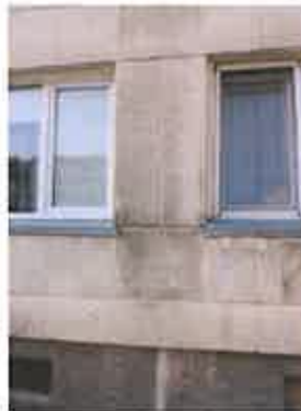
Figure 2. Place of sampling on facade
